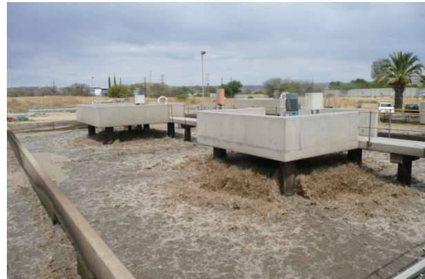
Field Trip: Waste water treatment plant
